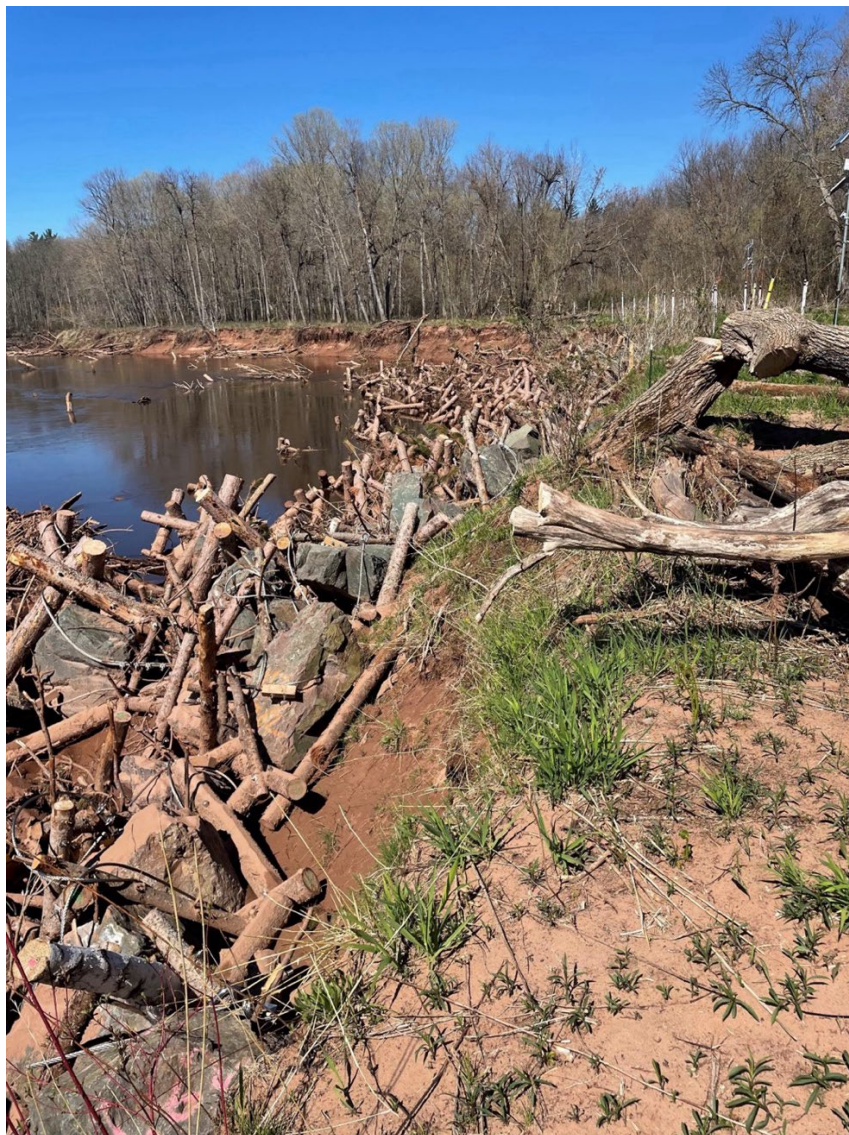
Figure 1: The Log Jacks from the Upstream End (May 8, 2025)
