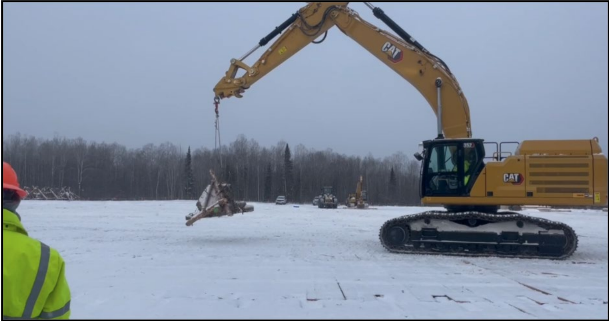
Fig. 12. Lift Test of Small Log Jack at Staging Area
