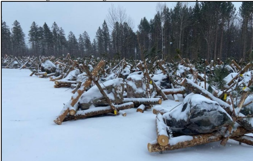
Fig. 8. Finished Log Jacks at Off-Site Assembly Area
