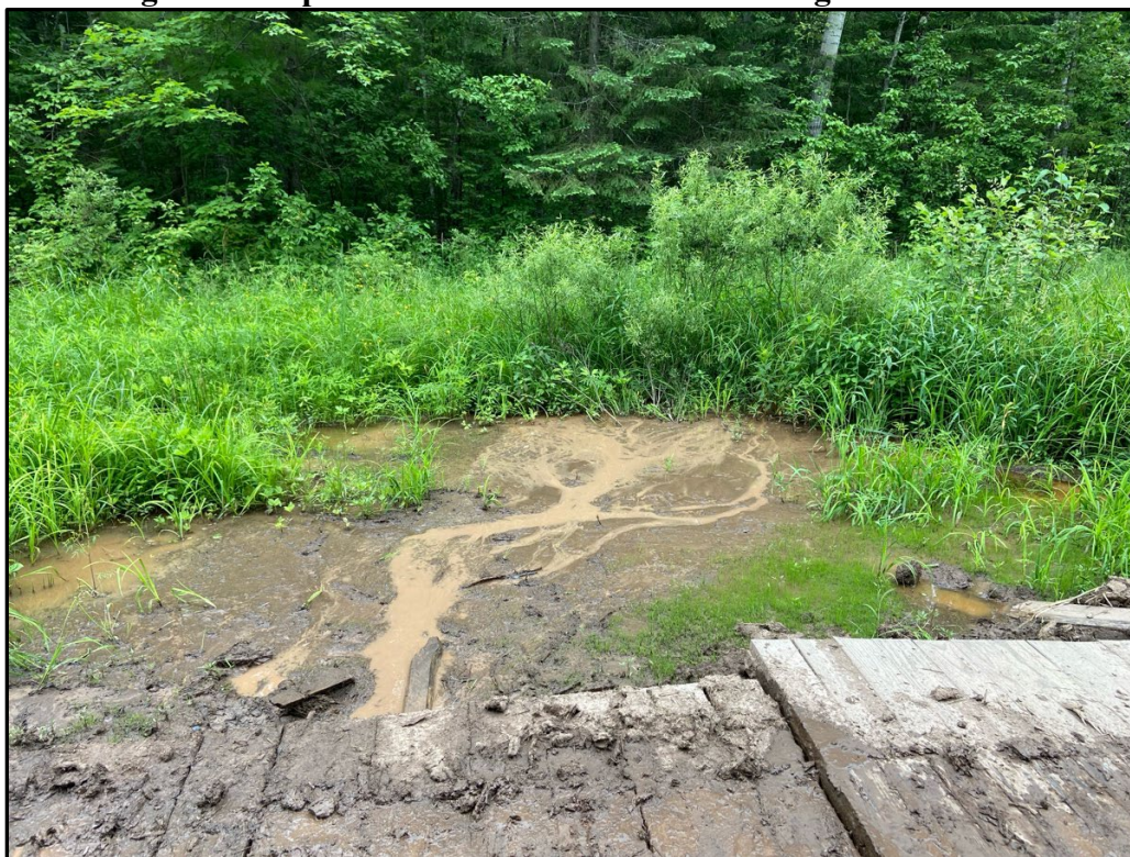
Fig. 4: Example of Watercourse Pollution Along Access Route
