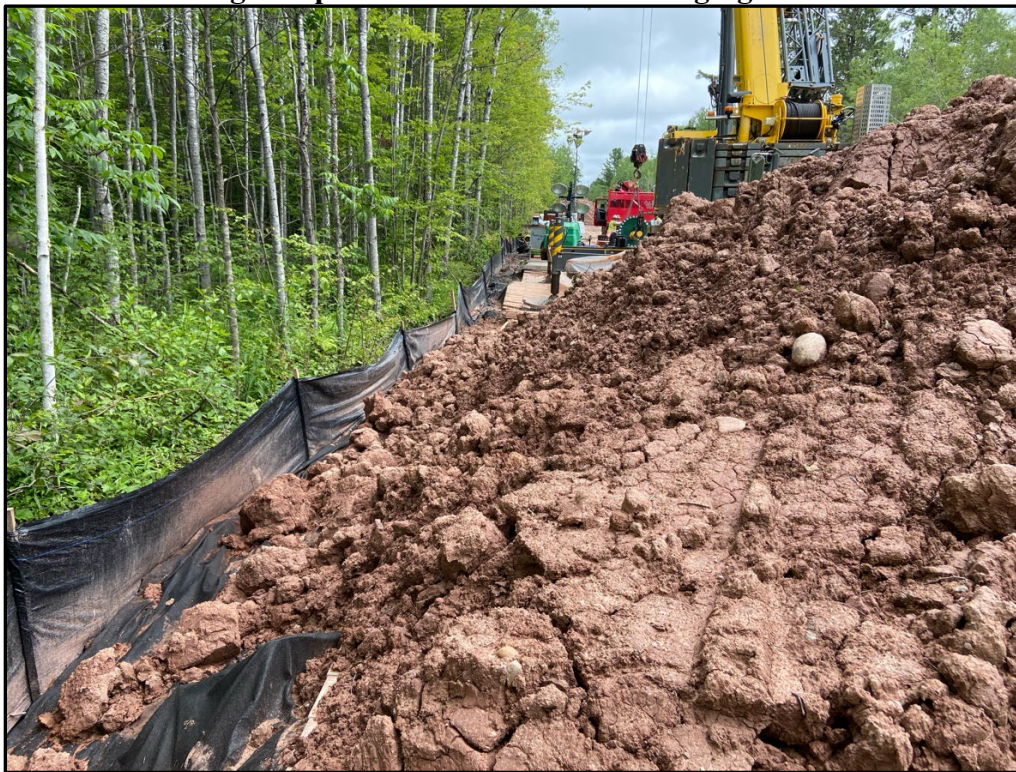
Fig. 7: Spoil Pile at Check Valve Staging Area
