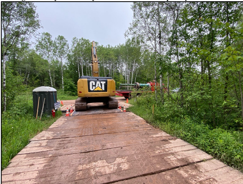
Fig. 2: Heavy Machinery on Check Valve Temporary Access Road
