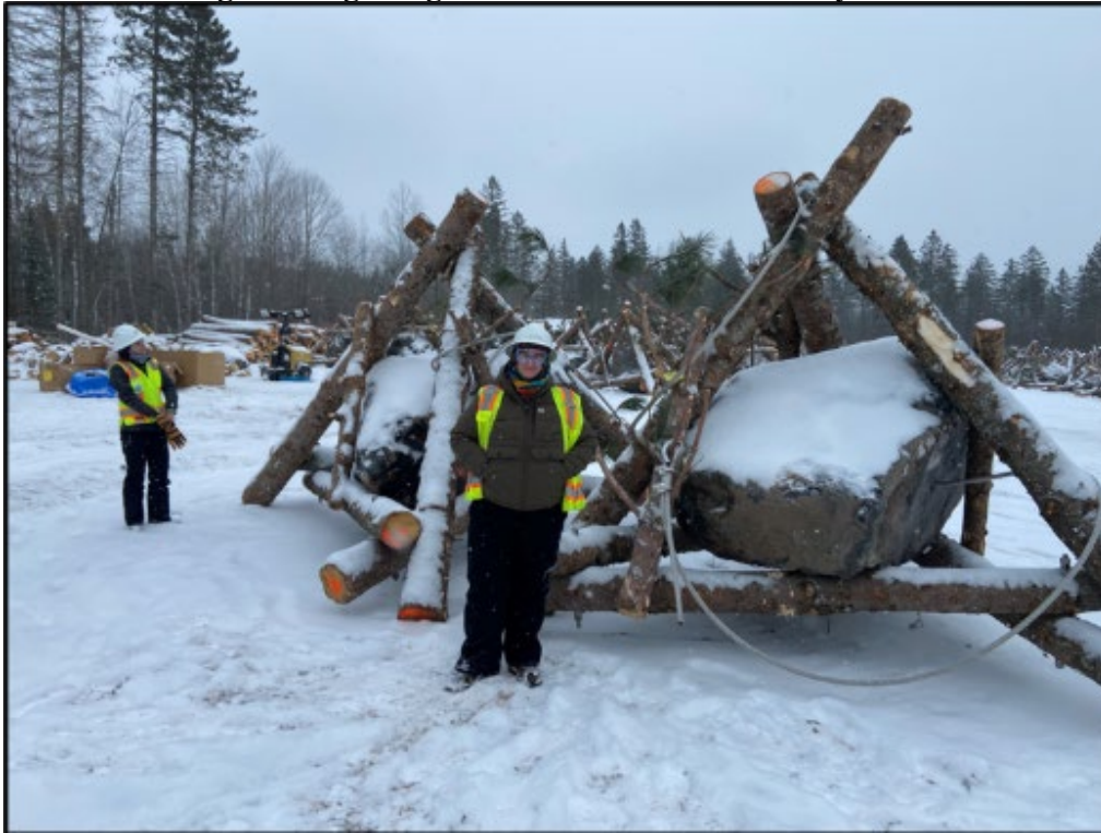
Fig. 9. Large Log Jacks at Off-Site Assembly Area
