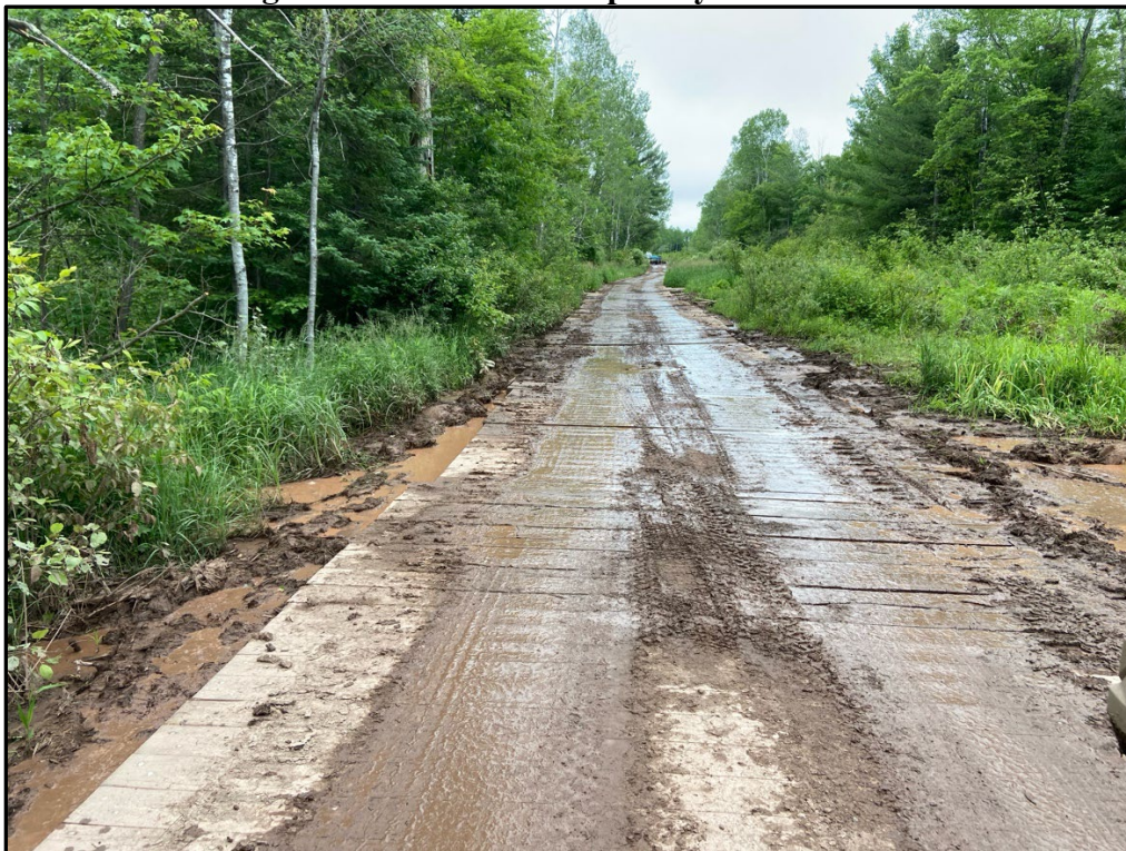
Fig. 1: Check Valve Temporary Access Road
