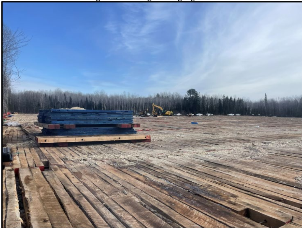
Fig. 11. Matting of Staging Area
