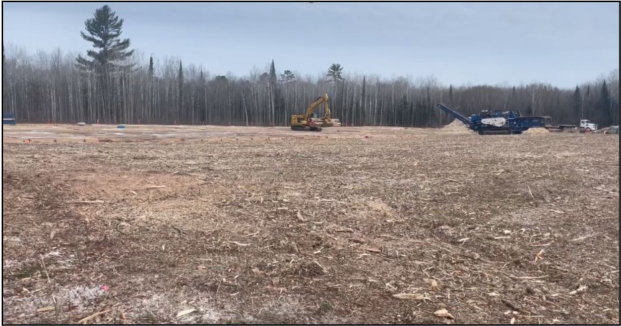
Fig. 10. Clearing and Chipping of Timber and Vegetation at Staging Area
