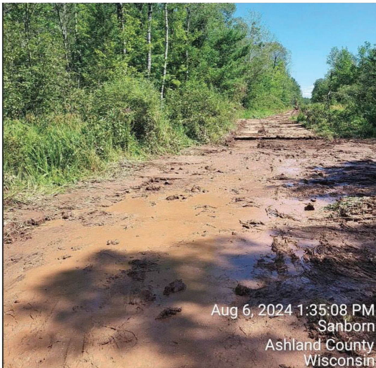
Figure 8. The photo shows the condition of the wetlands along the access route immediately after construction matting was removed. As you can see in the photo, the limits of soil disturbance are wider than the construction matting (see the width of construction matting in the background of the image).
