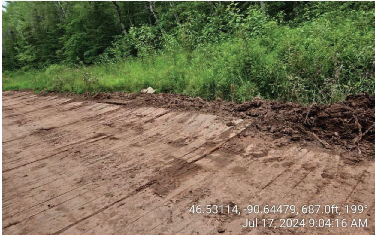
Figure 7. Soils are being pushed out from under the construction matting at drier areas along the access road (as compared to Figure 6) as soft topsoil is displaced from construction matting, which is supposed to be “protective” of the underlying landscape.
