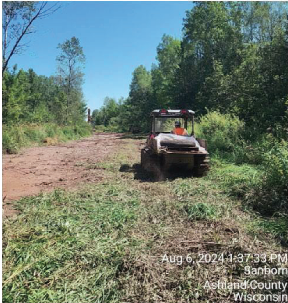
Figure 2. Photo from August 6, 2024, showing an Enbridge crew member operating a tracked vehicle off of the construction matting. The construction matting was placed in the muddy area shown on the left side of the photo—in the background, you can see the excavator that is picking up the construction matting as the Enbridge crew demobilizes from the site.
