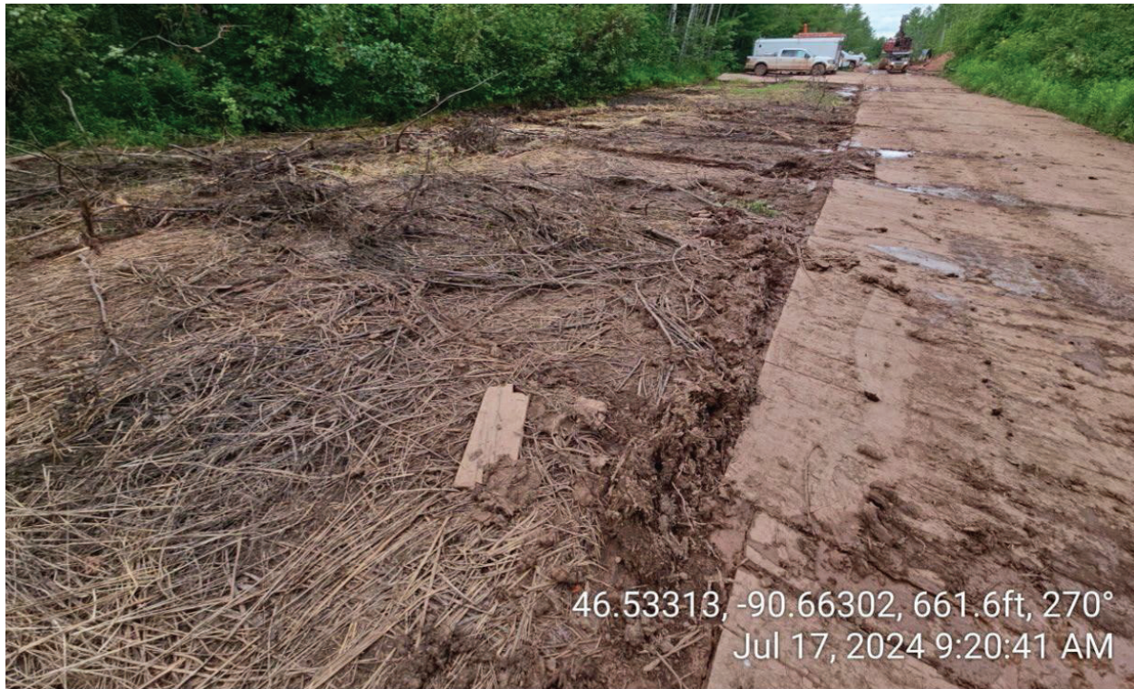
Figure 12. A photo from July 17, 2024, showing a location where timber matting was installed, then removed, for construction activities on the Reservation on Line 5.
