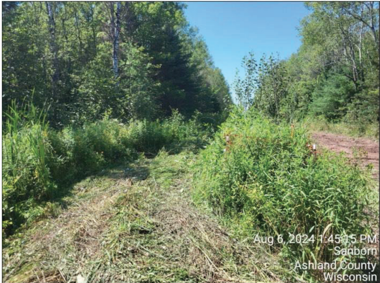
Figure 3. Areas of orange fencing were only installed around the culturally important plants that Enbridge was required to protect per tribal and federal permits when the plants were located within 5 feet of the construction matting. The lack of the orange construction fencing was not indicative of the lack of the protected plants, which were found at multiple locations along the corridor. The photo shows where Enbridge contractors drove around the fenced area (left side of the photo) instead of remaining on the construction matting, which would have been placed on the right side of the photo.
