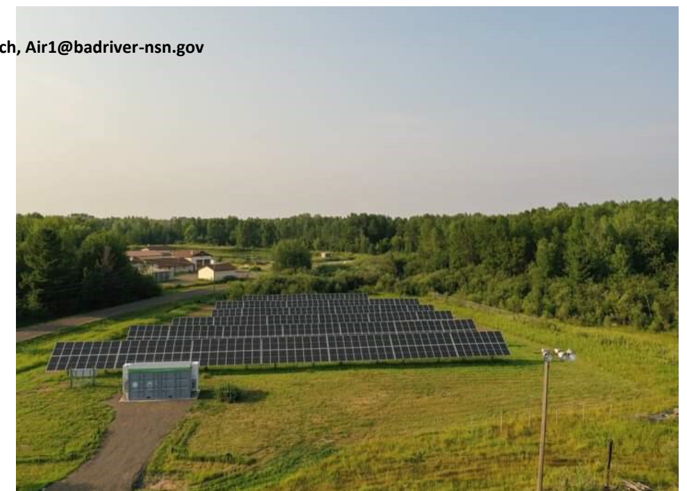
Picture 1: Wastewater Treatment Plant Microgrid- Battery Storage is located directly in front followed by the solar array and WWTP building in the back.
