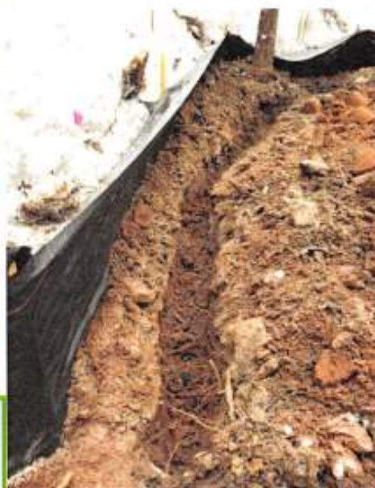
Figure 3: Groundwater interception trench greater than 14 inches deep.
