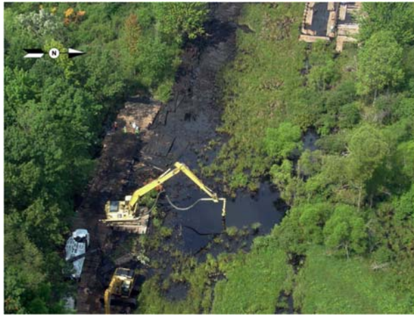
Vacuum truck on wooden matting near Line 6B spill, 2010
